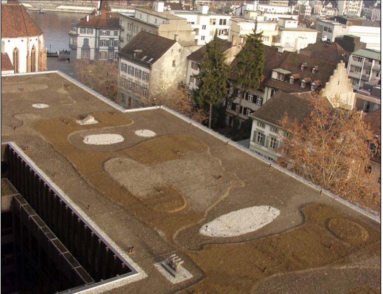
Figure 2: Newly constructed green roof on the Klinikum 2 of the Cantonal Hospital of Basel, built in accordance with the city's new guidelines on green roofs and urban biodiversity. (Photo: Stephan Brenneisen)
