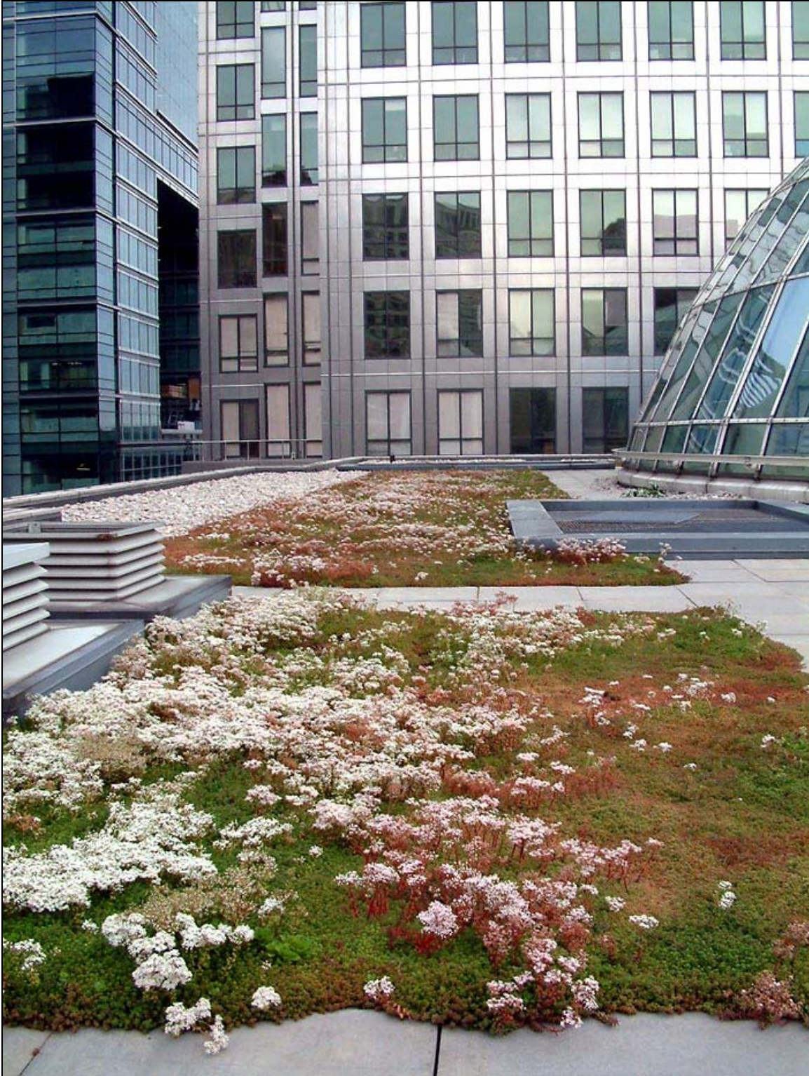
Figure 1: Retail Sedum roof, Canary Wharf, London.
