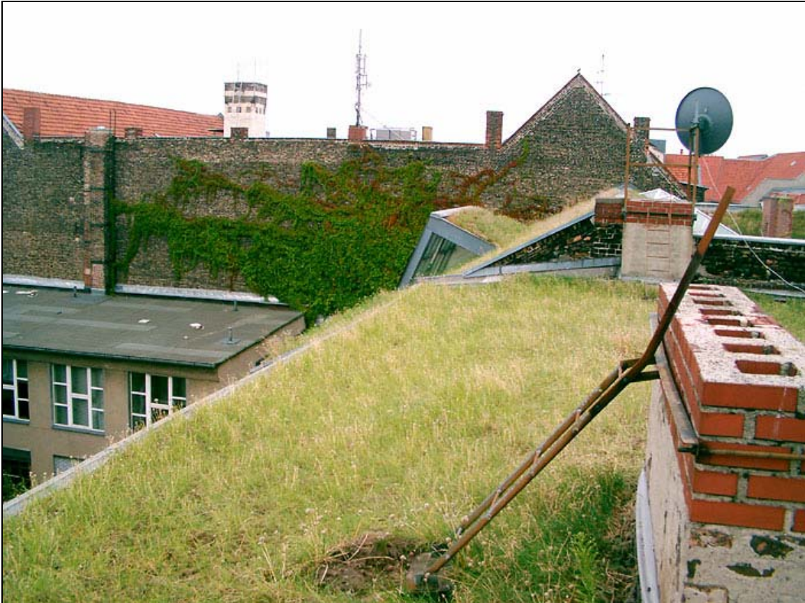
Figure 1a: The PLU research site in Berlin-Kreuzberg. In the foreground is flat sub-roof 9, which had the highest plant diversity of all the 10 sub-roofs in this project. The north-pitched sub-roof 10 is visible in the background; it had the lowest plant diversity.
